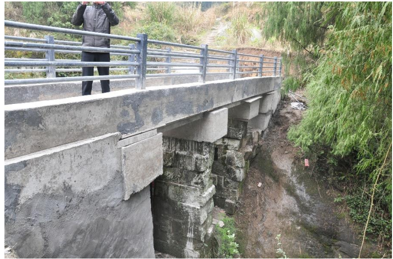
NO.279 堰沟湾过水桥 (已竣工)
